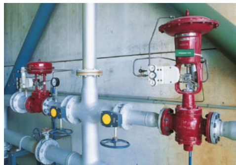
Deployment of NOVATEC® Premium in a salt extraction plant
